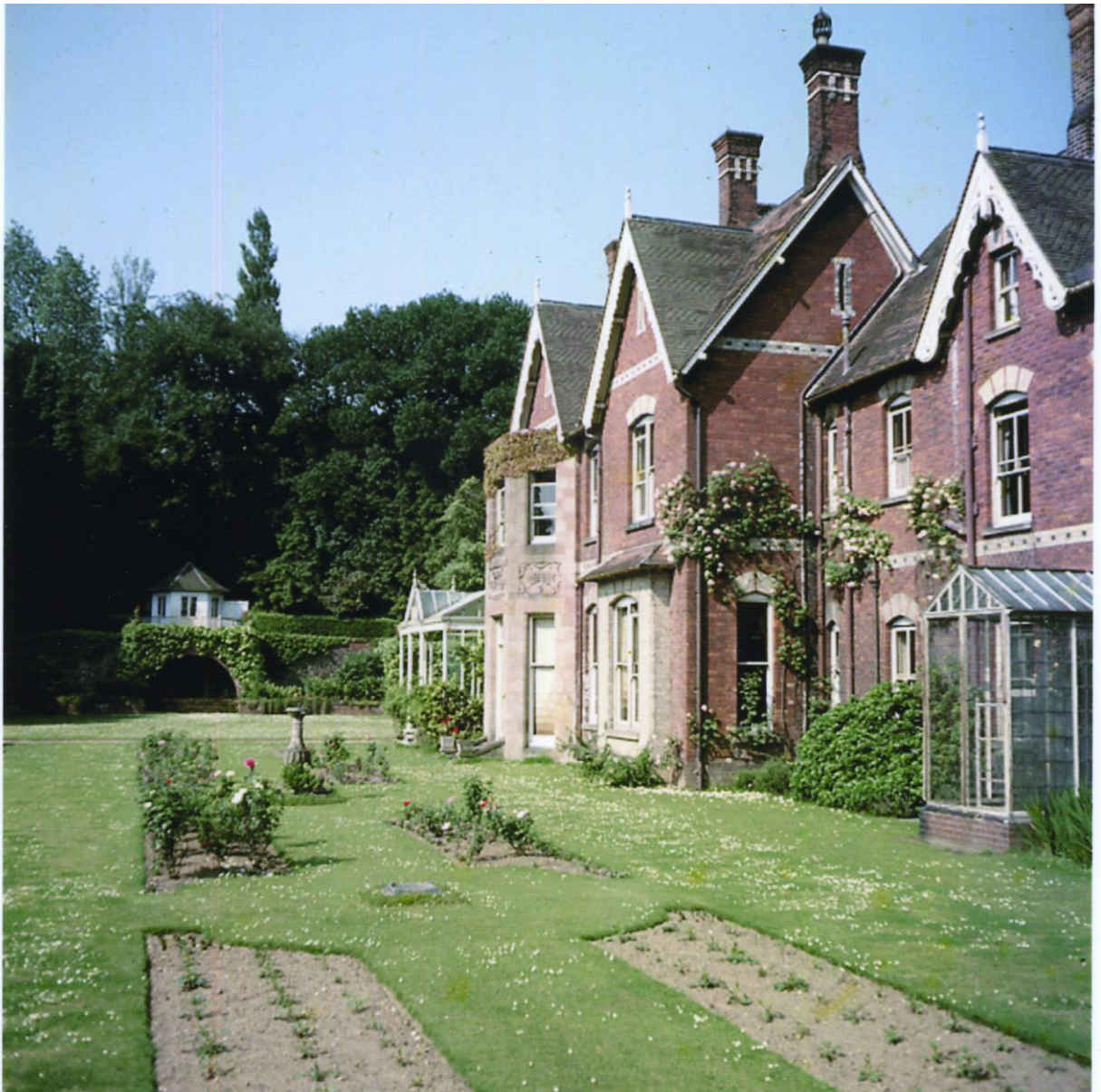
Broomfield - South aspect looking west (1955)
