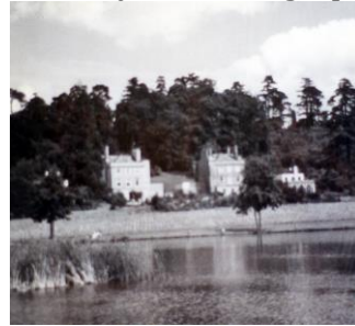
After the fire c1946
